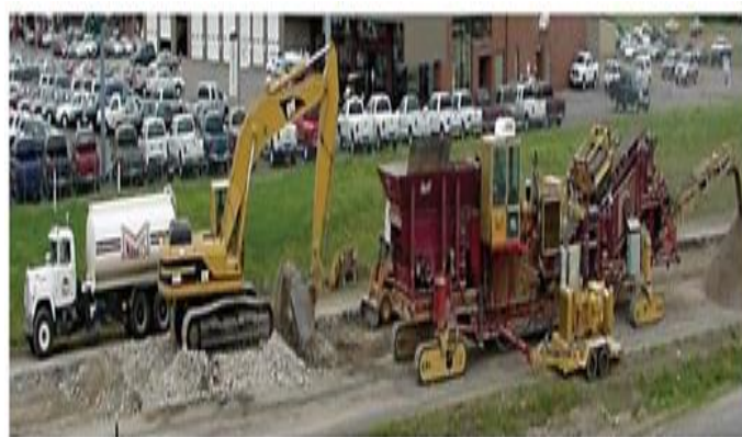
Fig. 2. In-situ recycling of mobile concrete pavement.
